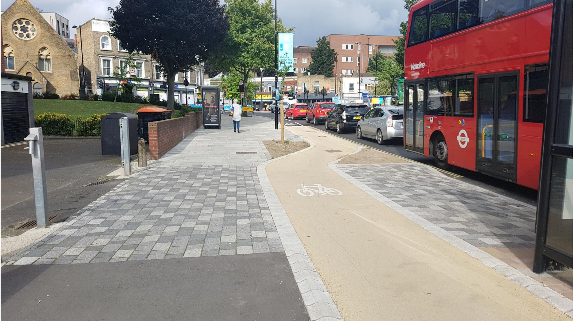
View of one of Wick Road's new segregated cycle tracks, installed as part of changes that reintroduced two-way traffic to the road. The changes are aimed at improving cycle permeability and access to the Olympic Park.
